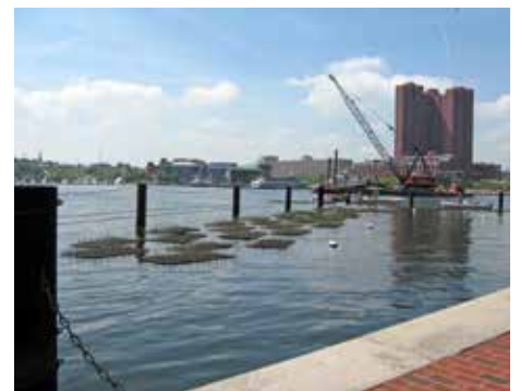
Floating wetlands being deployed in Baltimore's Inner Harbor, Maryland. Photo © Caroline Wicks, IAN Image Library
