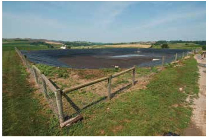
The lagoon holds liquid waste used for fertilizer after the solids have been separated by an anaerobic digester to produce energy. Photo © U.S. Department of Agriculture.
