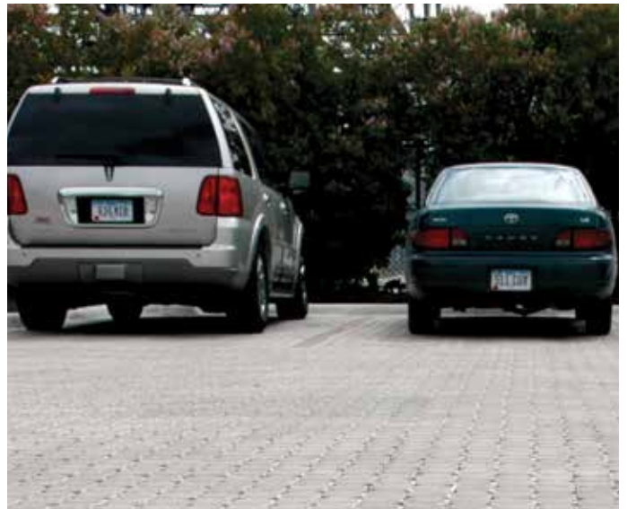
Modular paver blocks serve as a pervious paving system in a commercial parking lot. This practice allows for stormwater to infiltrate into limestone and underlying soils instead of directly into storm sewers. Photo © Jason Johnson, USDA Natural Resources Conservation Service.
