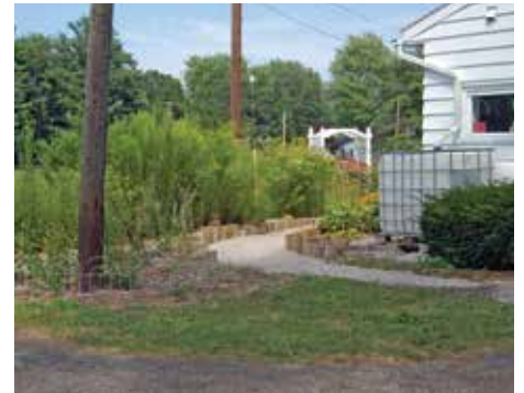
A rain garden and rain barrel used simultaneously for collection and filtration of stormwater runoff. Photo © Alexandra Fries, IAN Image Library
