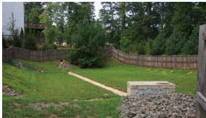
A stormwater drainage basin in a residential backyard directs excess, untreated runoff to the subsurface soil where it can filter naturally through the soil. Photos © Tim Auer, USGS.
