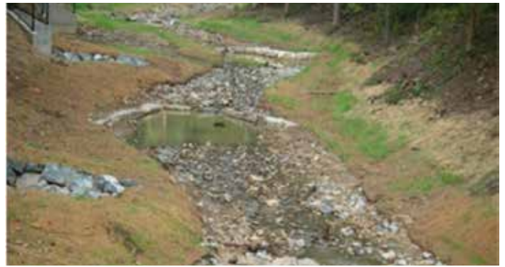
A constructed wetland site at Stony Run in north central Baltimore was used to assess whether constructed wetlands could be effective at reducing nitrate-N. Photo © Melanie Harrison, NOAA.
