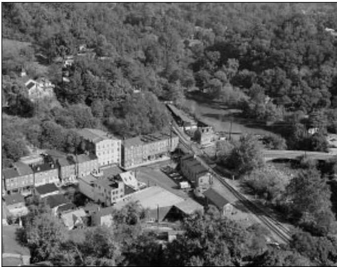
Figure 96: Aerial View of Ellicott Mills Looking North Toward Ellicott City, Maryland.
