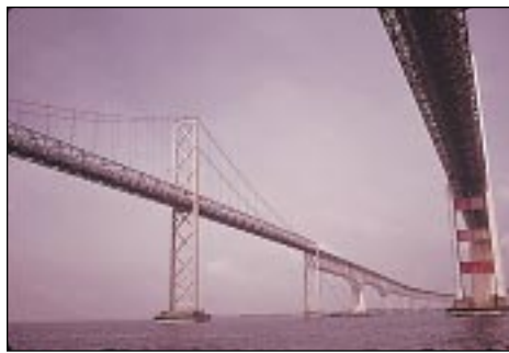
Figure 108: Chesapeake Bay Bridges, June, 1973. (Photograph courtesy of the U.S. Environmental Protection Agency and the National Archives)
