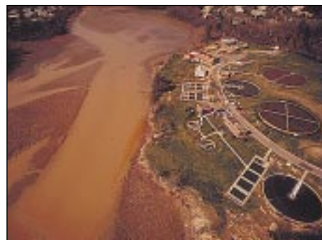
Figure 114: Water Filtration Plant, Occoquan, Virginia, 1973.
