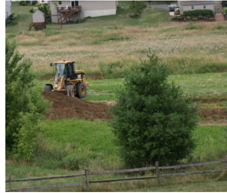
Sediment removal from the forebay of the water quality wetland in 2008.
