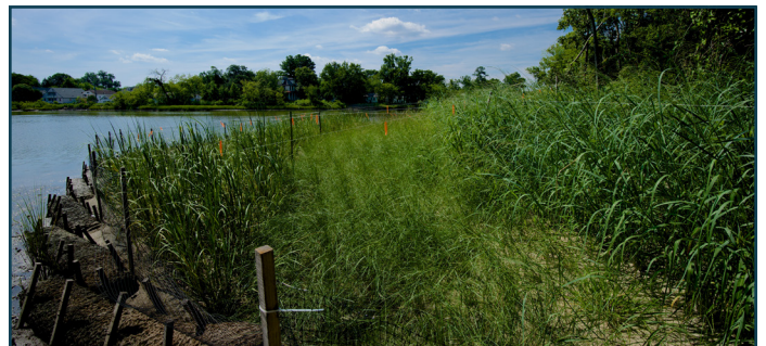
An urban tidal wetland project in Norfolk, Virginia uses coconut fiber logs for temporary erosion control.
