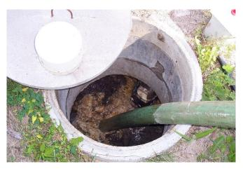
Figure S-1-1. Pumping sludge out of a septic tank, a routine part of septic system maintenance. Source: MCPA Flickr. (<u>https://flic.kr/p/UScorM</u>).
