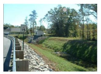
Figure D-13-2. Dry detention basin. Source: Simpson and Weammert-Lane Report (p. 201).
