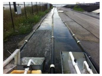
Figure N-3-1. Looking down the Maryland Port's Algal Turf Scrubber flow-way – the 2014 winner for the Most Innovative BMP in the Bay Award. Source: Chesapeake Stormwater Network.
