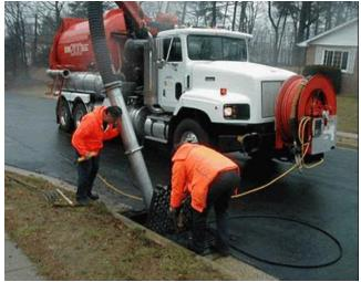
Figure D-10-1. Storm Drain Cleaning in Anne Arundel County. Work is completed on a rotating basis using a vactor (vacuum) truck to reduce sediment traveling to the Bay. Source: Anne Arundel County, Department of Public Works. <u>https://www.aacounty.org/departments/public-</u> works/highways/road-
