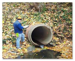
Figure D-8-1. Visual Inspections and Outfall Screening are used to look for any signs of flow discharges in storm drain manholes or outfalls. If found, samples are taken to measure flow, color, odor, oils, floatables, and water quality parameters. Source: Chesapeake Stormwater Network, Good Recipes for the Bay Pollution Diet U-6.
