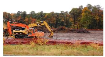
Figure D-3-2. Equipment rests on a construction site with stormwater barriers in place on Oct. 27, 2009. Source: Alicia Pimental/Chesapeake Bay Program.
