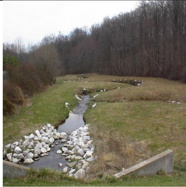
(a) Riparian Tree Loss Can be Severe During Construction unless Extreme Care is taken to Preserve and Protect Existing Trees
