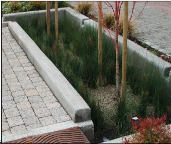
Figure 7 – Typical planter box (Source: Philadelphia Water Department, 2014)
