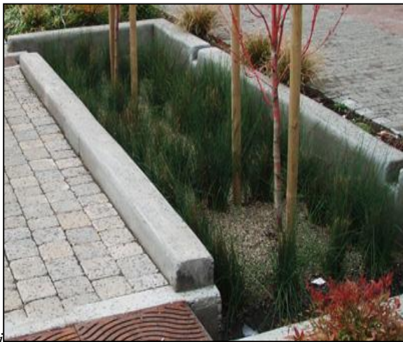
Figure 7 – Typical planter box (Source: Philadelphia Water Department, 2014)
