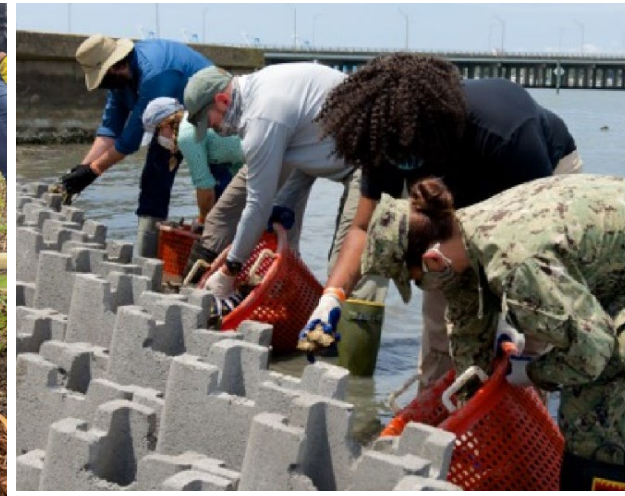
Naval Support Activity – Hampton Roads (VA) installing oyster castles along their shoreline
