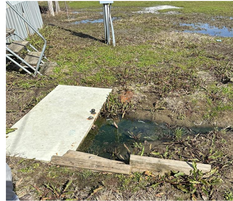
Image: Septic tank without lid, raw sewage on ground during Bolivar County, MS site visit.
