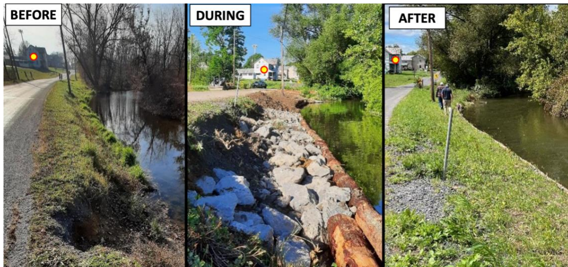
Figure 6. Union Creek Road project photo documenting installation of a 10 section mud sill to protect the road where a stream was threatening the road. Source: Pennsylvania Dirt, Gravel, and Low Volume Road Maintenance Program.
