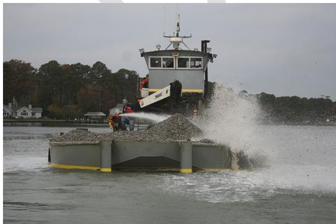
Contractors working for the U.S. Army Corps of Engineers, Norfolk District, use high-pressure water cannons to spread fossilized oyster shell in the Lynnhaven River in Virginia Beach, Va., in an effort to build medium relief oyster reefs for an ongoing oyster restoration project. (Photo courtesy USACE Norfolk)
