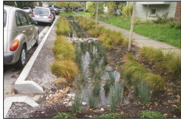
Figure 8 – Typical urban bioswale (Source: American Forests, 2012)
