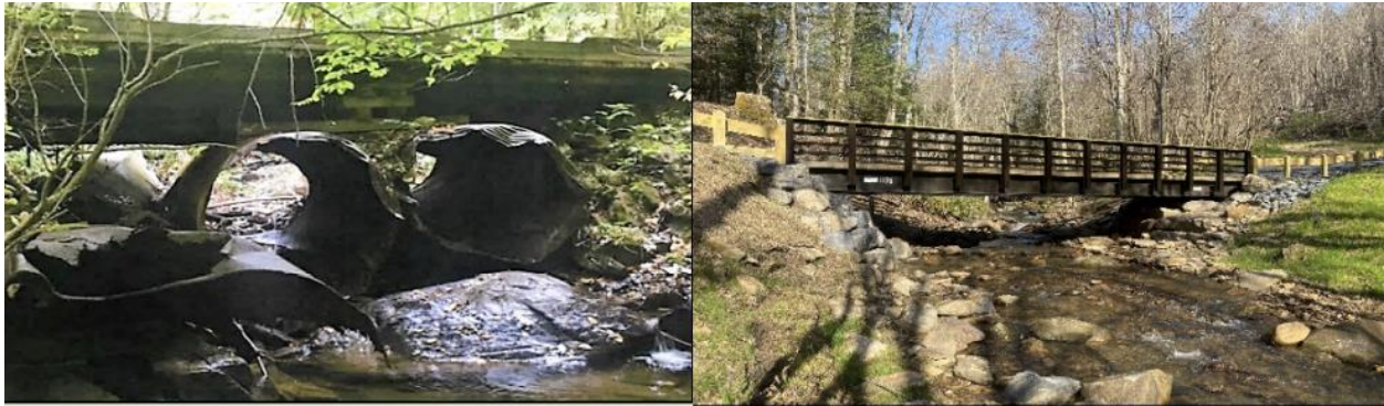
Figure 8. Wolfden Run road–stream crossing replacement near Kitzmiller, Maryland. Left: original multi-pipe culvert prior to replacement. Right: replacement span bridge following construction. Photo credit: Seth Moessinger, Trout Unlimited.
