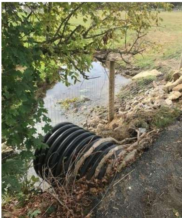
Figure 3. Outfall drop and scour pool at Site 2
