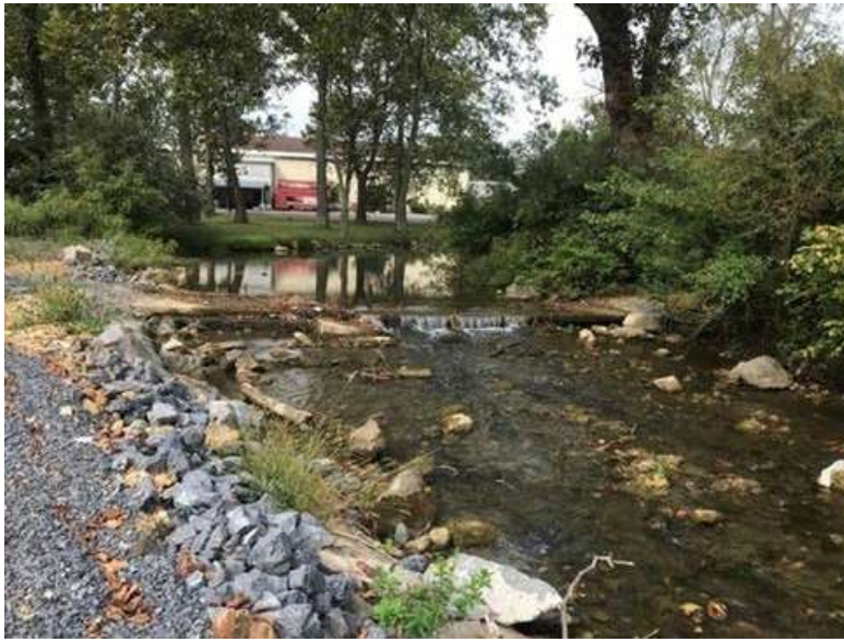
Figure 5. Low-water ford showing evidence of erosion at Site 4
