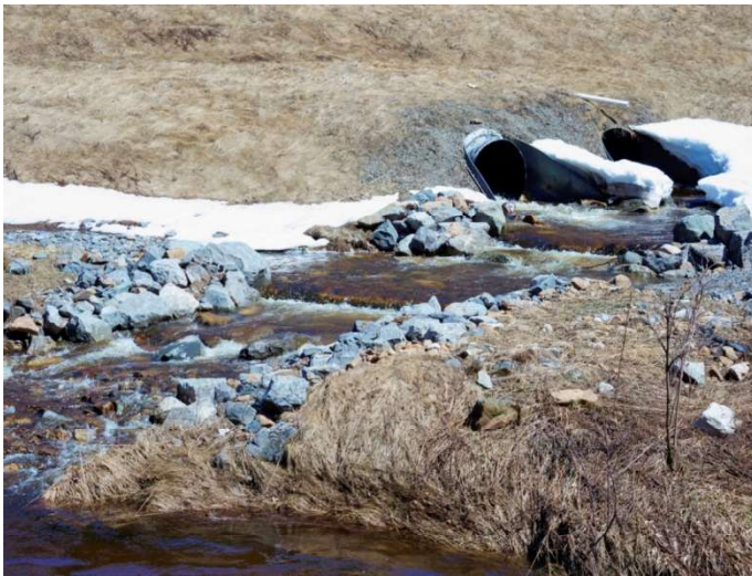
Figure 9. Steps and pools created to improve fish passage on Oats Run in Pocahontas County, WV
