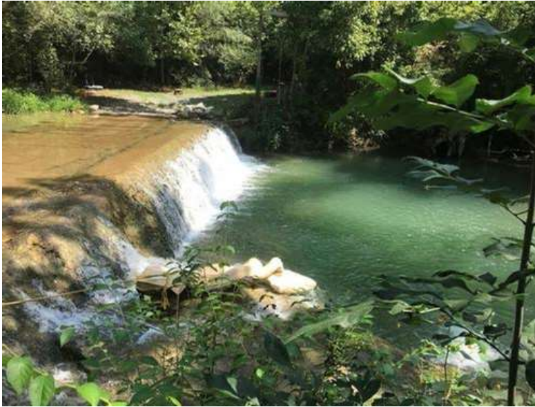
Figure 4. Barrier created by low-water ford at Site 3
