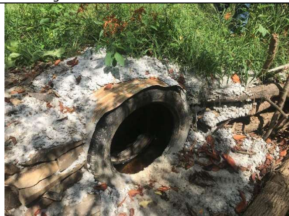
Mill Creek Headwaters: culvert constructed from tires, plywood, and concrete
