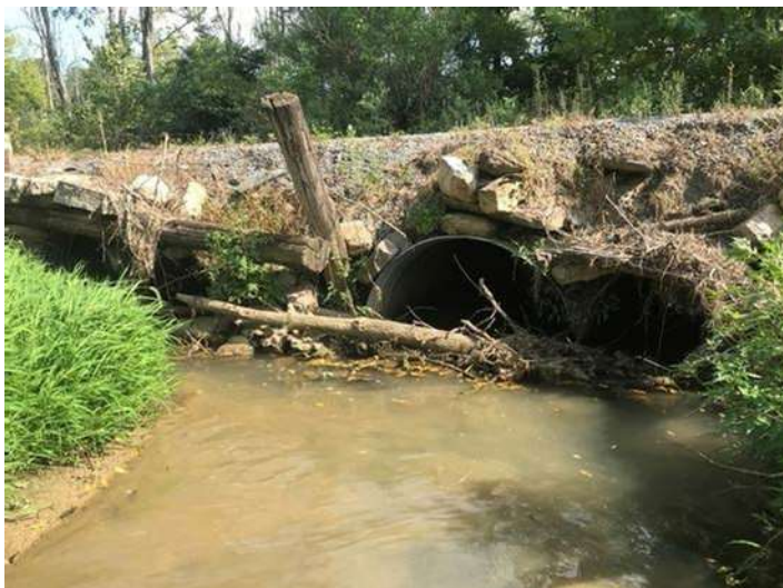
Figure 8. Evidence of debris jam at inlet of replacement implementation site
