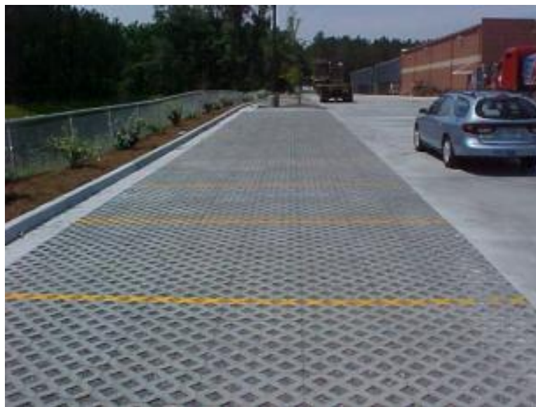
Figure B-6. Photo of Permeable Pavement in Good Condition
