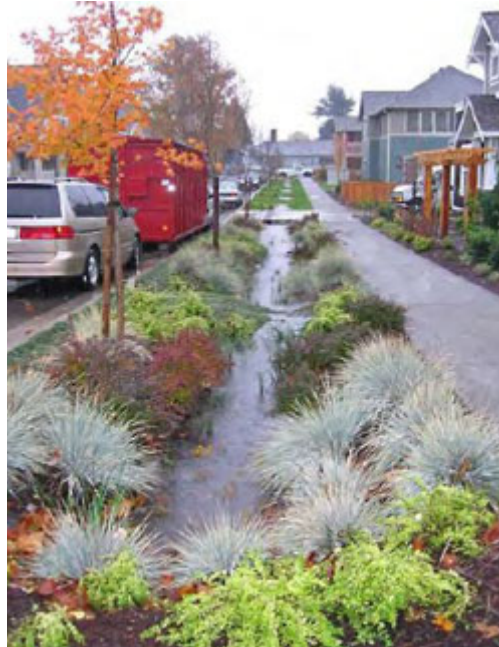
Water-filled planted swale during 25-year storm event
