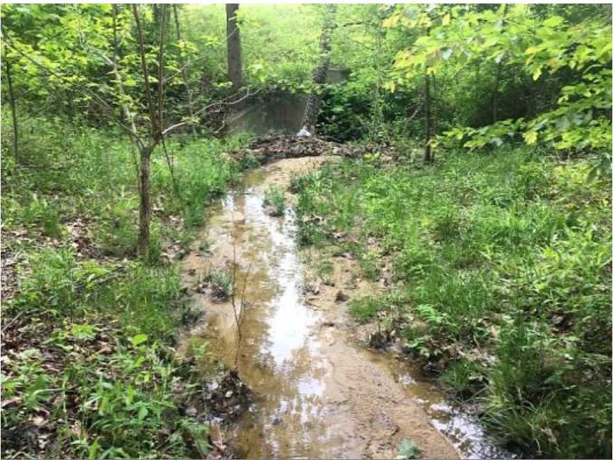
PRE- CONSTRUCTION: SAND GRAVEL DEPOSITION AT DOWNSTREAM CULVERT
