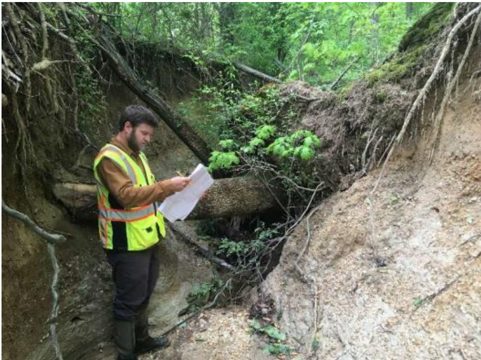
PRE – CONSTRUCTION: HIGHLY ENTRENCHED CHANNEL, BANK HEIGHT 7 FEET HIGH
