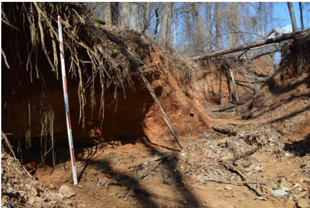
PRE - CONSTRUCTION: EXISTING, ENTRENCHED OUTFALL CHANNEL 2/29/2016
