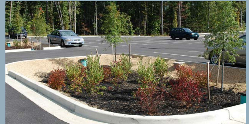
Above: An infiltration-based stormwater practice designed to intercept impervious surface runoff. (Photo courtesy of Chesapeake Bay Program)
