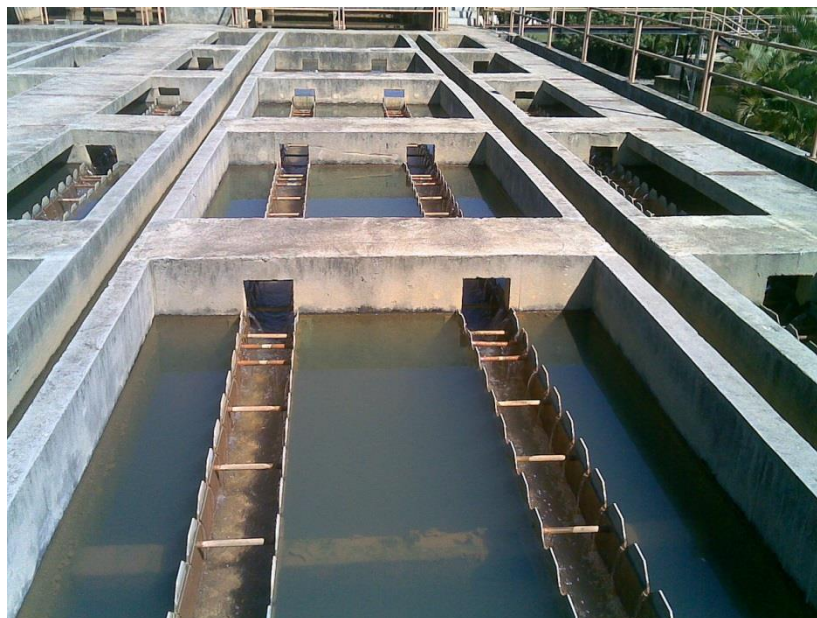
Figure STTL.1. Rectangular Clarifier (Wikipedia.org)
