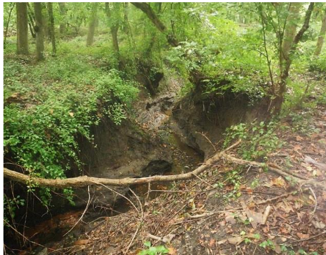
PRE - CONSTRUCTION: NEAR VERTICAL BANKS AND UNDERCUT TREES
