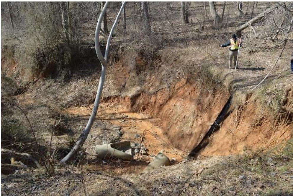
PRE-CONSTRUCTION: EXISTING ENTRENCHED OUTFALL CHANNEL ,
