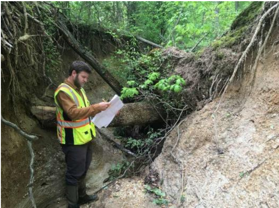
PRE – CONSTRUCTION: HIGHLY ENTRENCHED CHANNEL, BANK HEIGHT 7 FEET HIGH 5/18/2016
