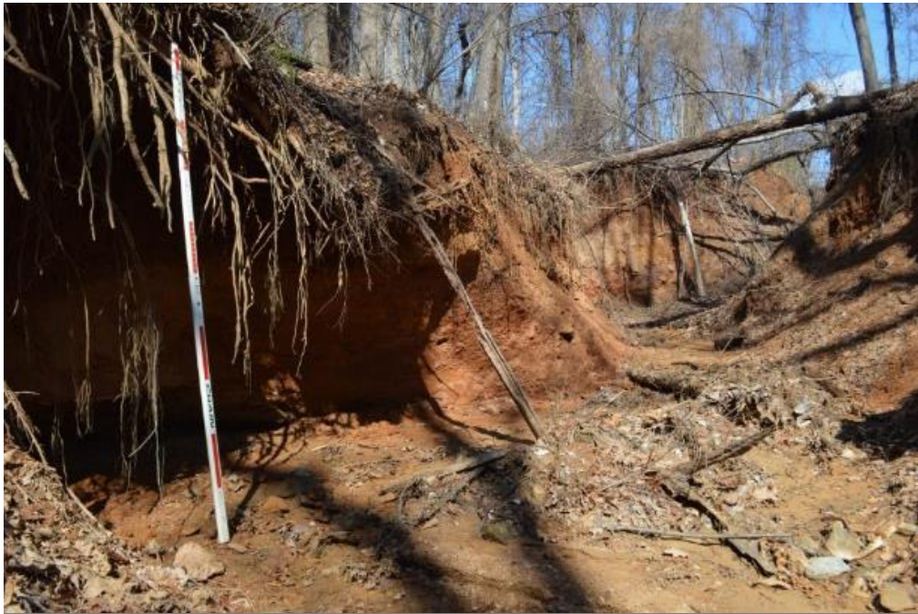
PRE - CONSTRUCTION: EXISTING, ENTRENCHED OUTFALL CHANNEL 2/29/2016
