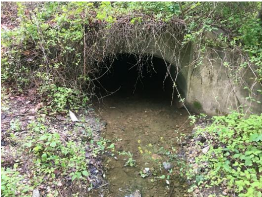
PRE - CONSTRUCTION: PIPE OUTFALL
