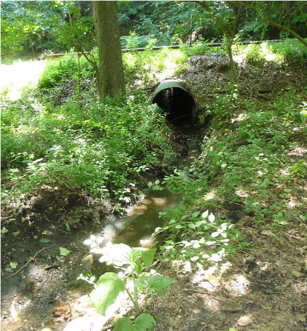
PRE-CONSTRUCTION: PIPE OUTFALL 6/27/2014
