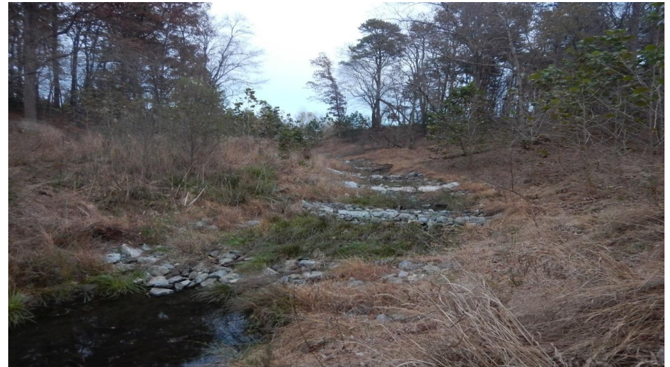
POST – CONSTRUCTION – LOOKING UPSTREAM 11/14/2018
