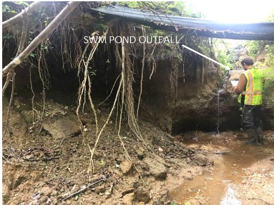
PRE - CONSTRUCTION: HEADCUT , LOOKING TOWARDS POND OUTFALL 5/18/2016
