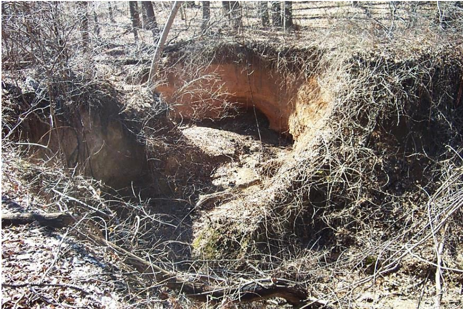
PRE - CONSTRUCTION: EXISTING ENTRENCHED OUTFALL CHANNEL,
