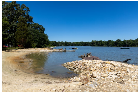
A living shoreline that replaced a bulkhead at West River United Methodist Center. (Photos by Ethan Weston/Chesapeake Bay Program)
