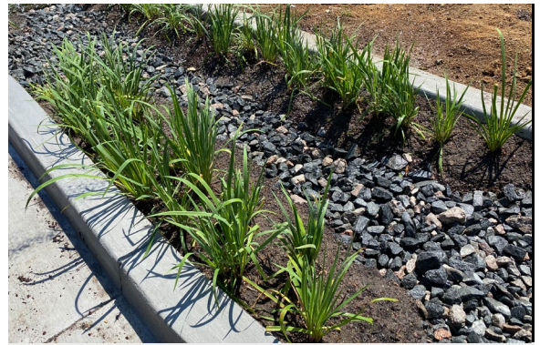
Rain garden helps reduce stormwater runoff in the surrounding area. (Photo: James River Association)
