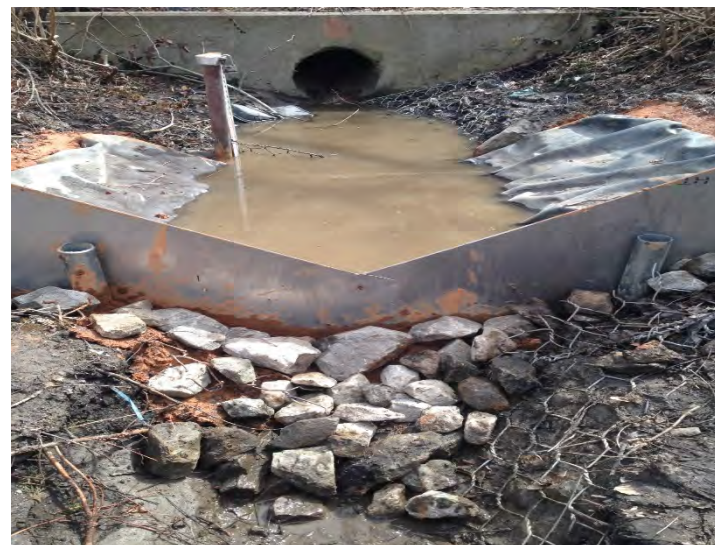
Glyndon: Inlet A immediately following weir installation
