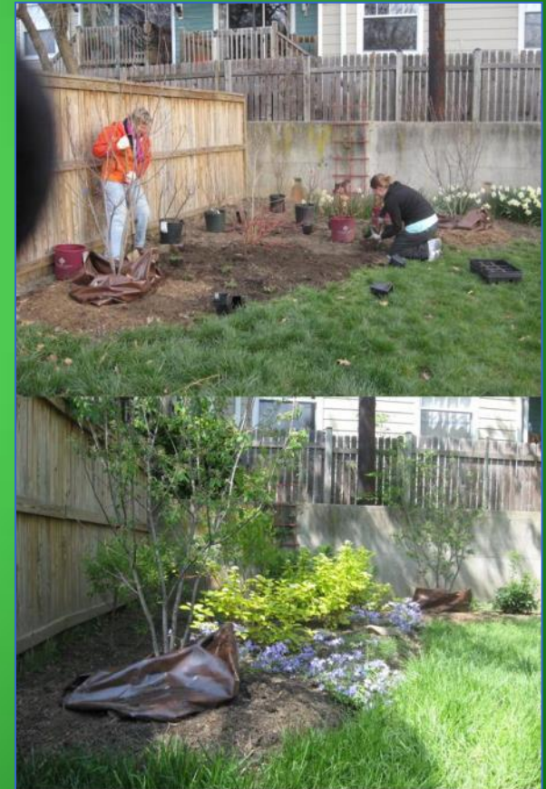
RiverSmart Home Installation Before & After Completion
