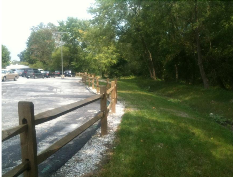
Figure B-4. Picture of a Filter Strip in Good Condition
