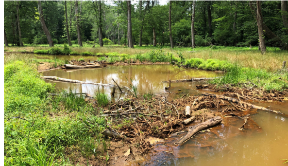
Figure 1. Floodplain Restoration Using Legacy Sediment Removal (Courtesy: Jeff Hartranft, PA DEP and Art Parola, University of Louisville)
