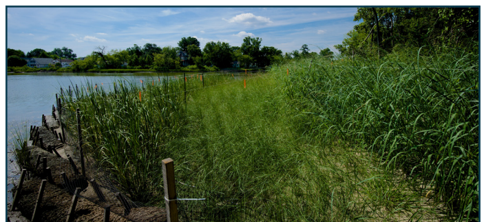
An urban tidal wetland project in Norfolk, Virginia uses coconut fiber logs for temporary erosion control.
