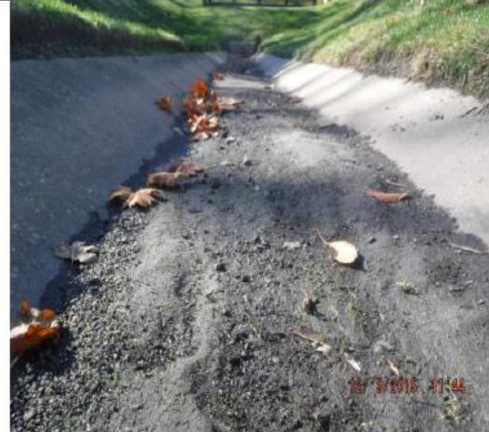
Loss of Capacity – Full Pilot Channel
