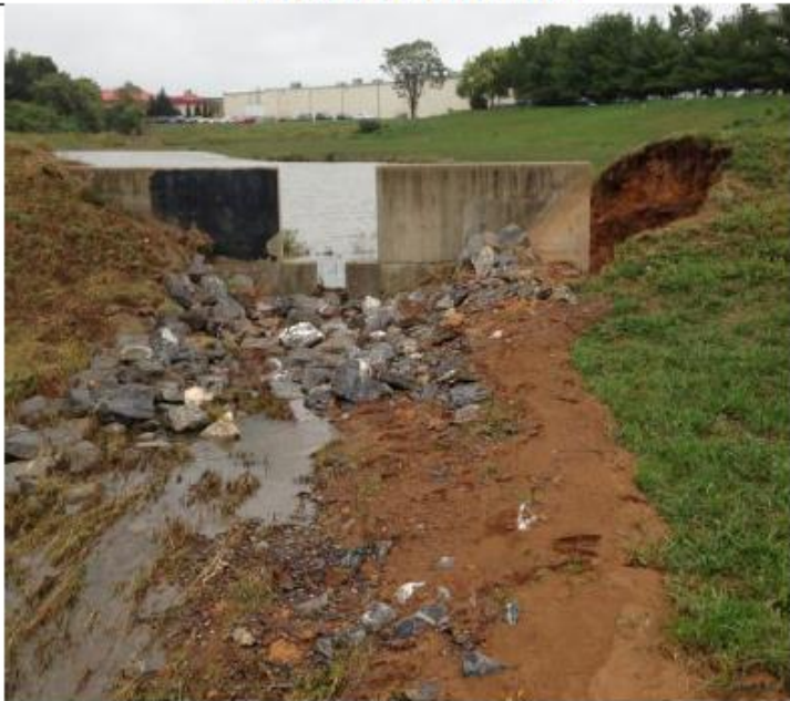
Embankment Failure
