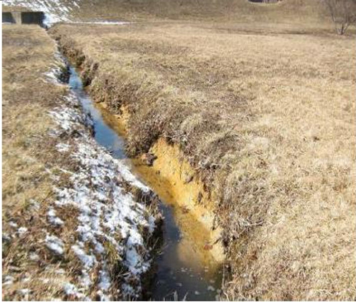
Erosion at the Inlet
