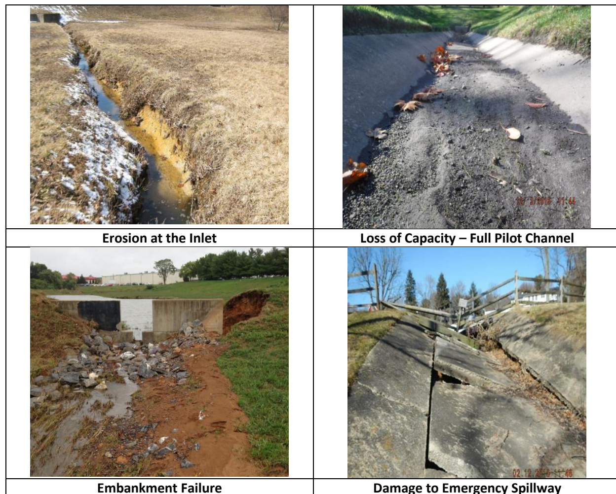
Figure 6. Examples of vulnerable design elements for stormwater ponds.
