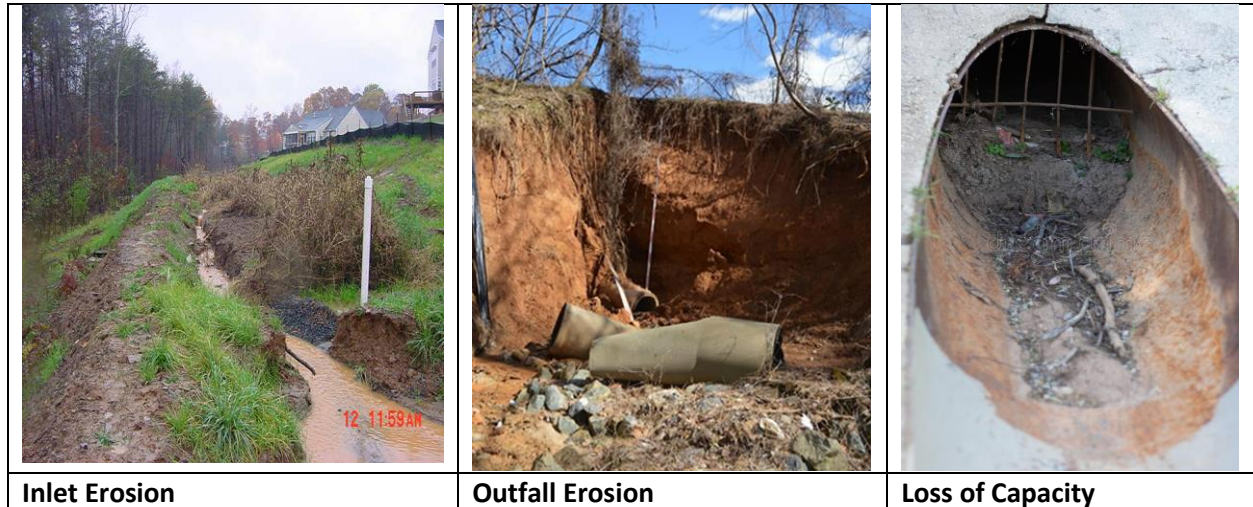
Figure 5. Examples of vulnerable design elements for conveyance practices.
