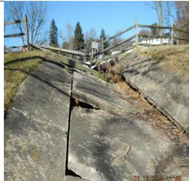
Damage to Emergency Spillway
